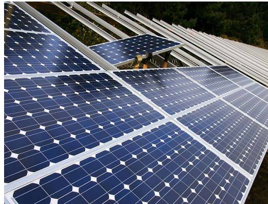
Image 17. Installation of solar panel | Source
