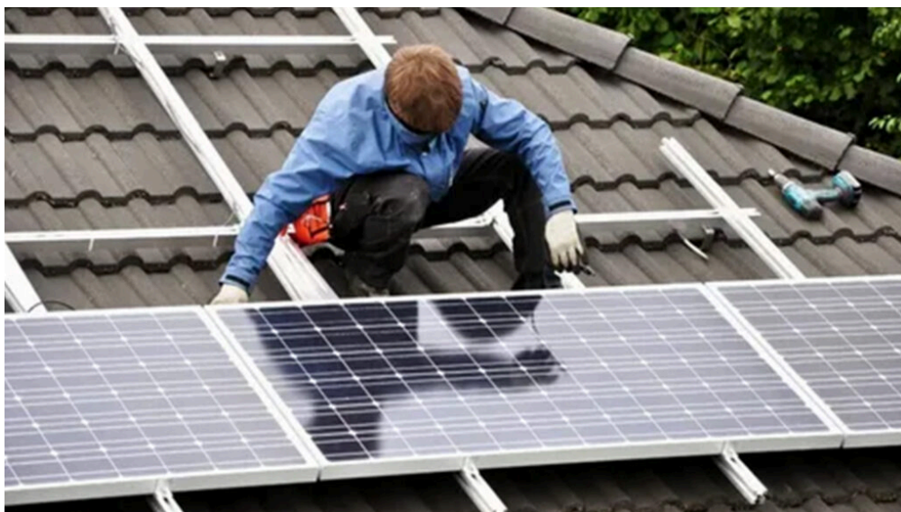
Fig 7.3 Rooftop solar MMS for sloped roof structures | Maysun solar
