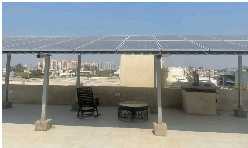
Fig 7.2 Elevated Mounting structures | RK Solar Energy
