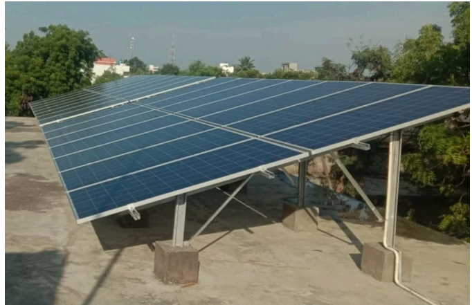
Fig 7.1 Rooftop Solar MMS for RCC roof : Ballast mounted and Anchored system | GRENGY SOLAR
