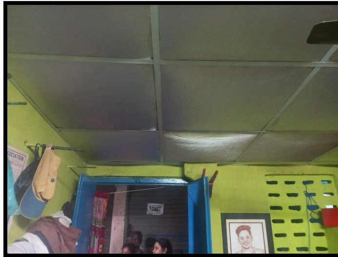
Installed alufoil static mechanism mounted on aluminium channel support
