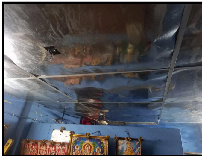
Galvanized iron sheet with insulation, after installation
