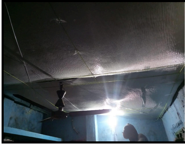
Installed alufoil static mechanism mounted on steel wire support
