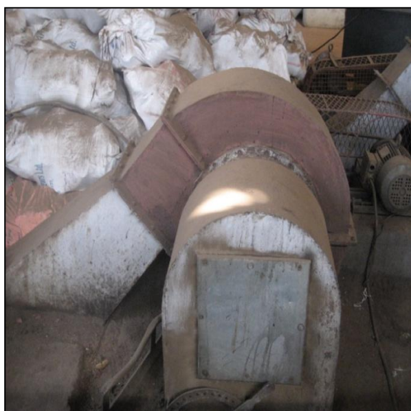
Fig 10.4 : ID Fan for Flue Gas Exhaust and Chimney | CAG
